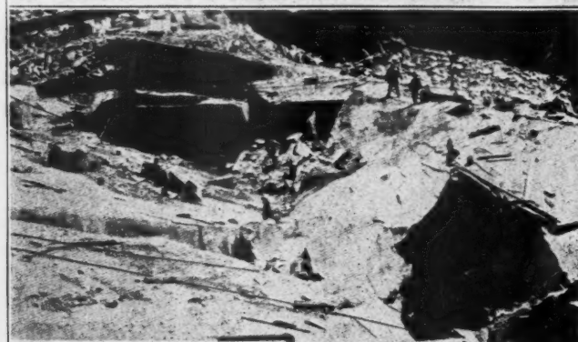
Another Big Sheet Ready for Service
